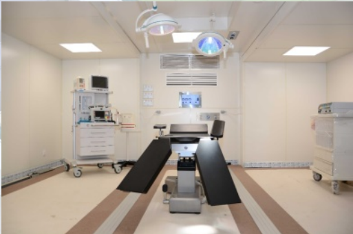
Surgical UNITS have medical gasses (O2, N2, vacuum), hygenic air-conditioning, ventilation with hepa filtration
