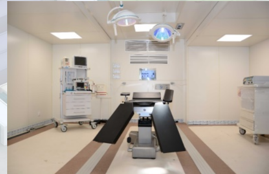
Surgical UNITS have medical gasses (O2, N2, vacuum), hygenic air-conditioning, ventilation with hepa filtration
