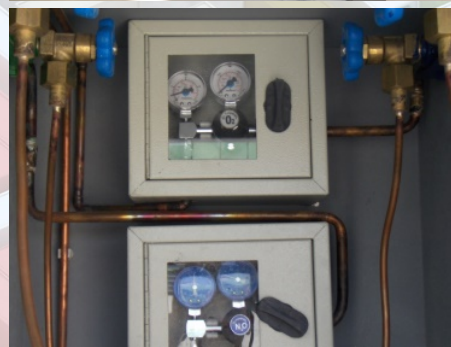
Surgical UNITS have medical gasses (O2, N2, vacuum), hygenic air-conditioning, ventilation with hepa filtration
